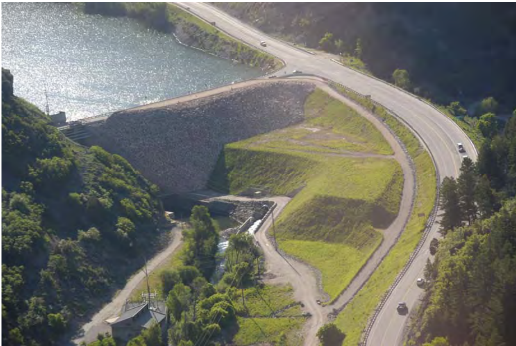
Figure 4.5.7-3. Pineview Dam (near Ogden, Utah). View showing stability berm to improve performance of the dam during a seismic event.
