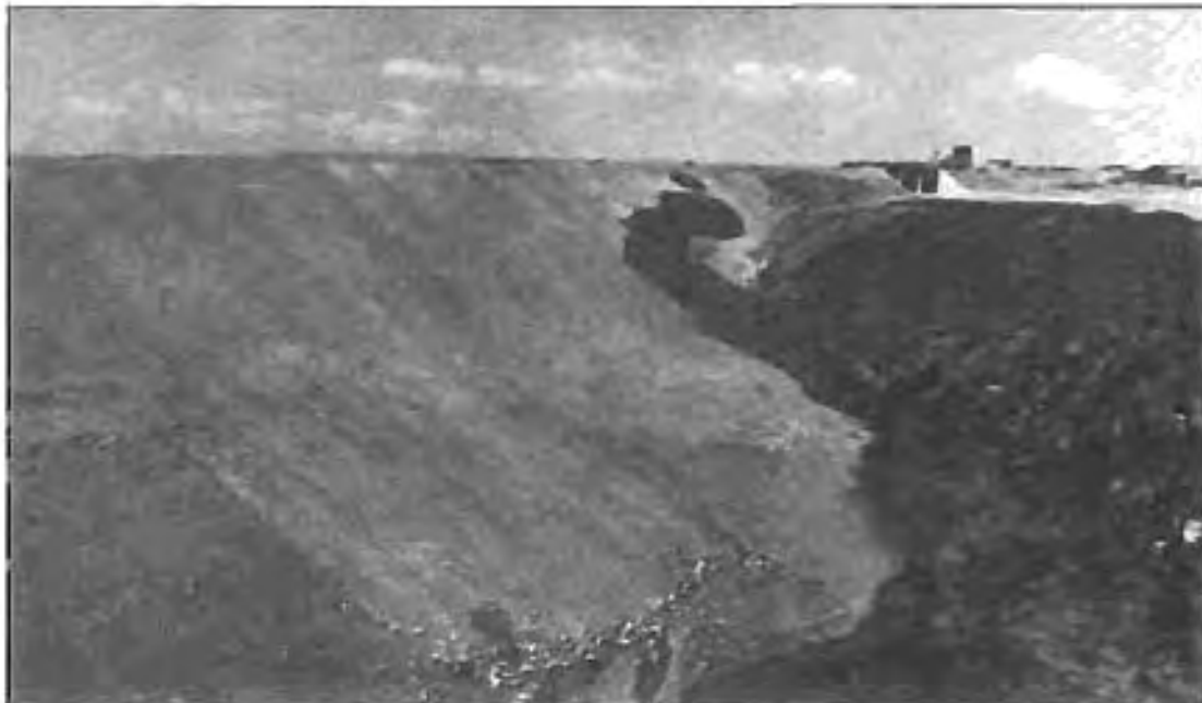
FIGURE 3. Development of erosion tunnel through Teton Dam. (USBR photo.)
