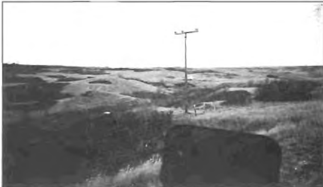
FIGURE 6. Landslide topography downstream of Gardiner Dam.
